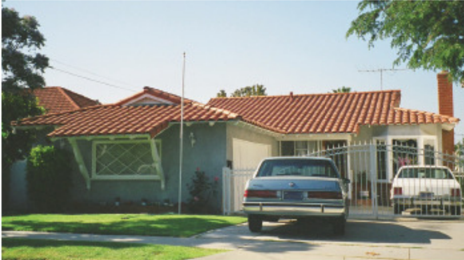
Figure 2-7 Typical one-story slab-on-grade house (from ATC, 2002).
