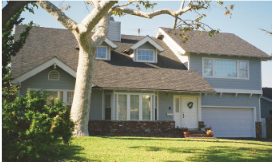
Figure 2-18 Split-level house, where the section of flooring above the garage is at a lower level than the main second-floor level (from ATC, 2002).
