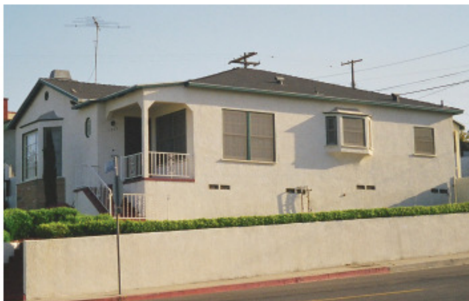
Figure 2-3 Typical one-story cripple-wall crawl-space house (from ATC, 2002).
